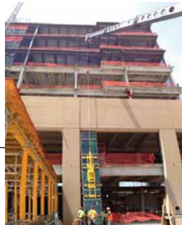
The first piece of glass is installed.
